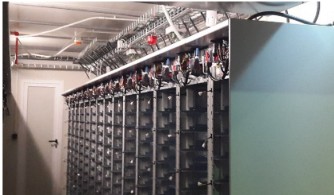
Figure 5: 40ft Containerized BESS
