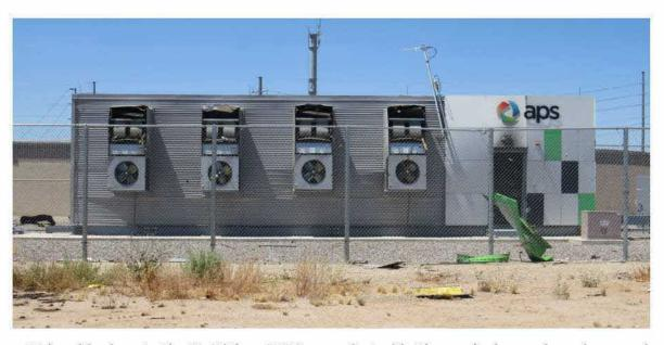
Figure 7 The side door to the McMicken BESS was ejected in the explosion and can be seen laying against the fence in the foreground
