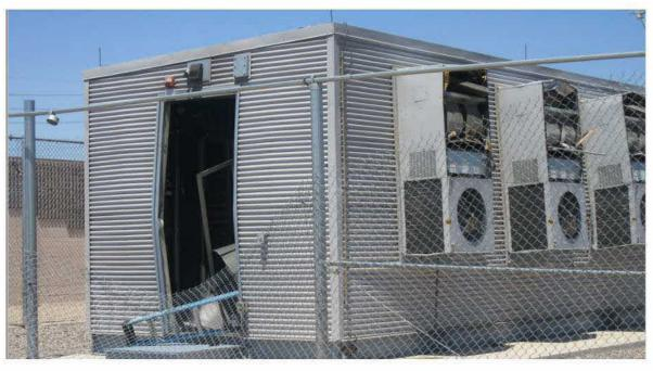
Figure 6 Damage to the rear door and HVAC systems of the McMicken BESS
