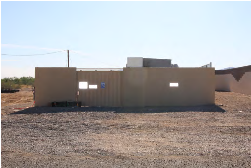
Figure 4.2: Photograph of the solid wall and gate to the northeast of the ESS [13].
