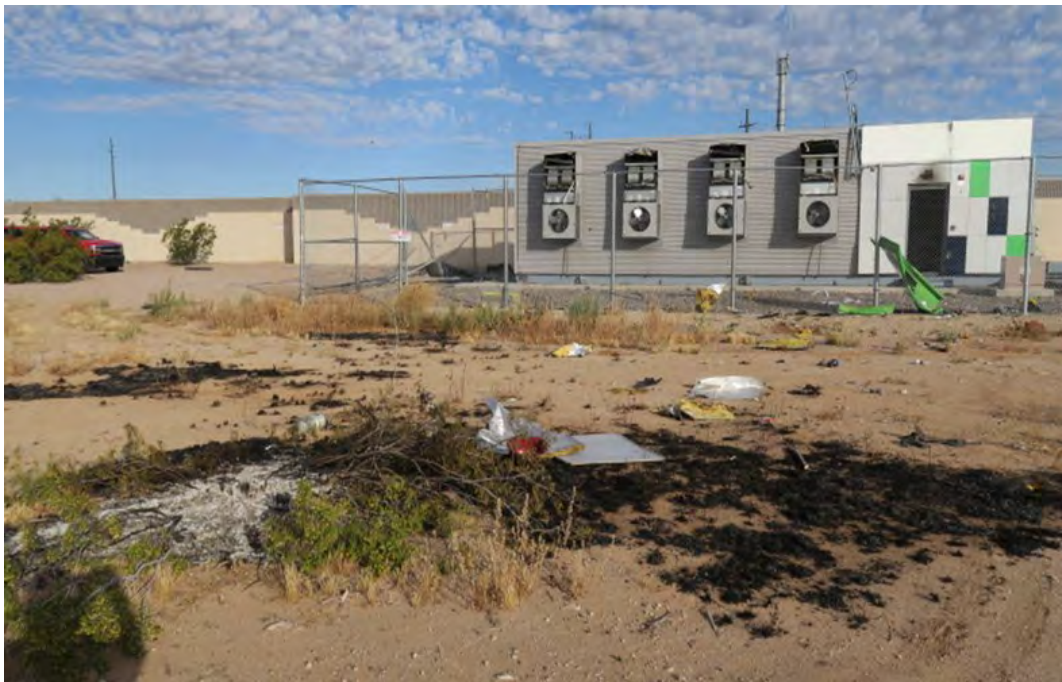
Figure 4.19: Photograph of burned bush, E193 Capt's helmet, and SCBA tank removed during the deflagration [6].
